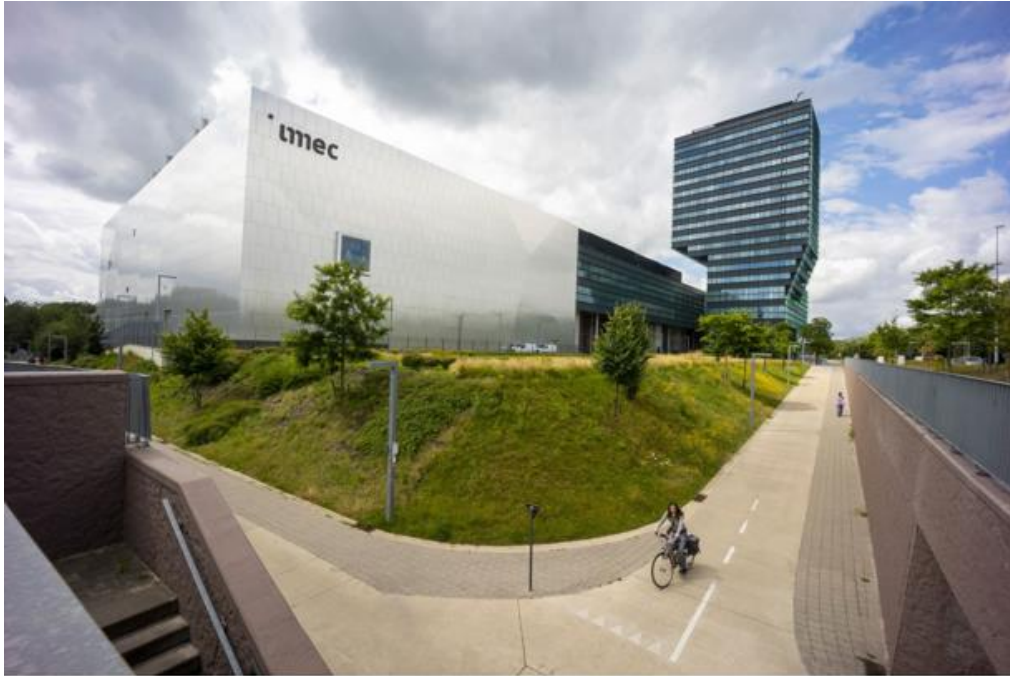
The imec R&D center and tower in Leuven, Belgium. Photographer: Olivier Matthys/Bloomberg
